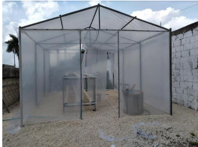
Figure 8. Final external structure of the hydroponic greenhouse prototype.
